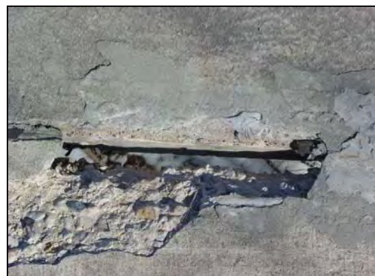
An example of a hole in the concrete of the pedestrian bridge
