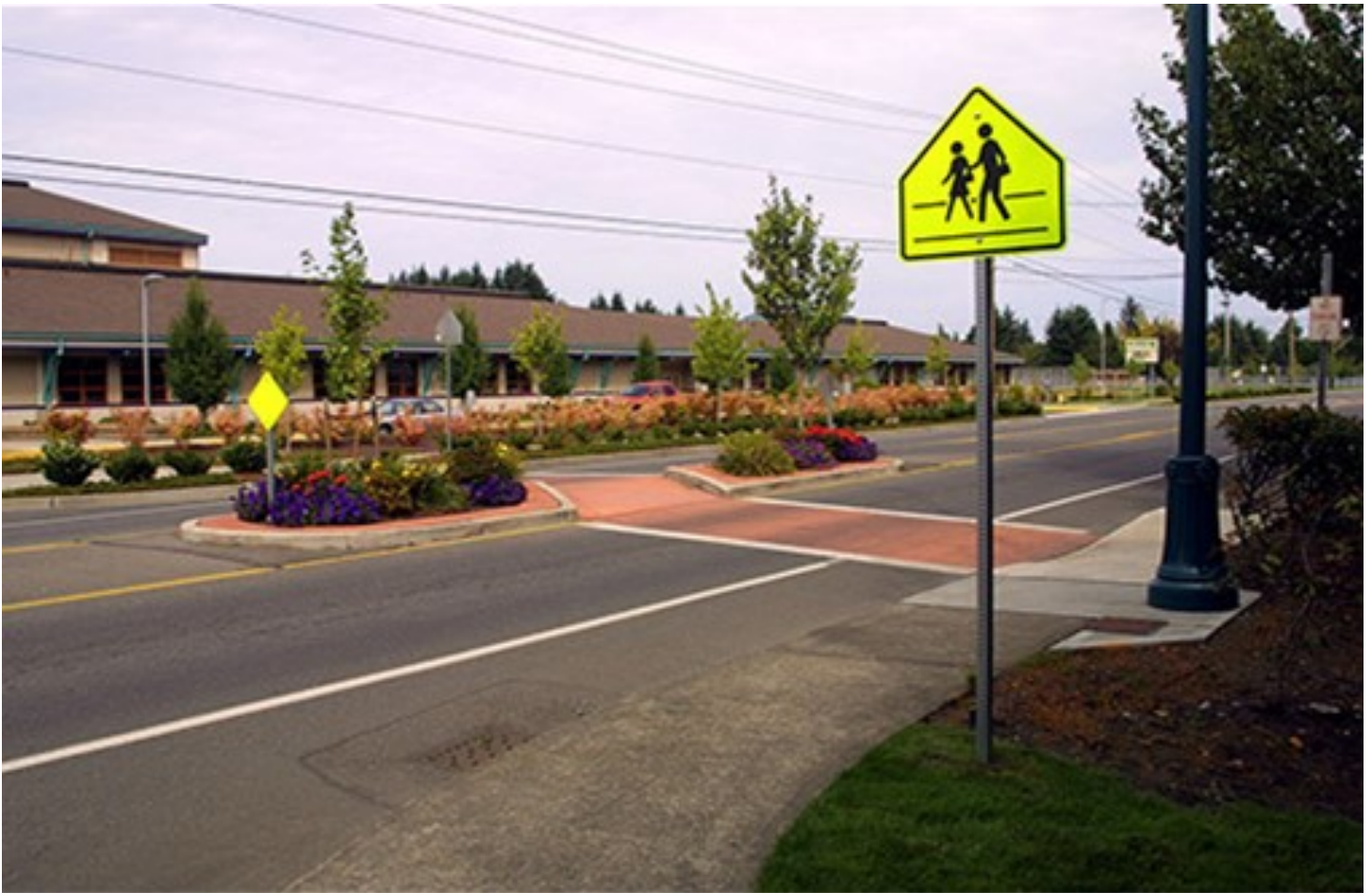
Staggering the crosswalks allows pedestrians to view the oncoming lane before continuing across.
