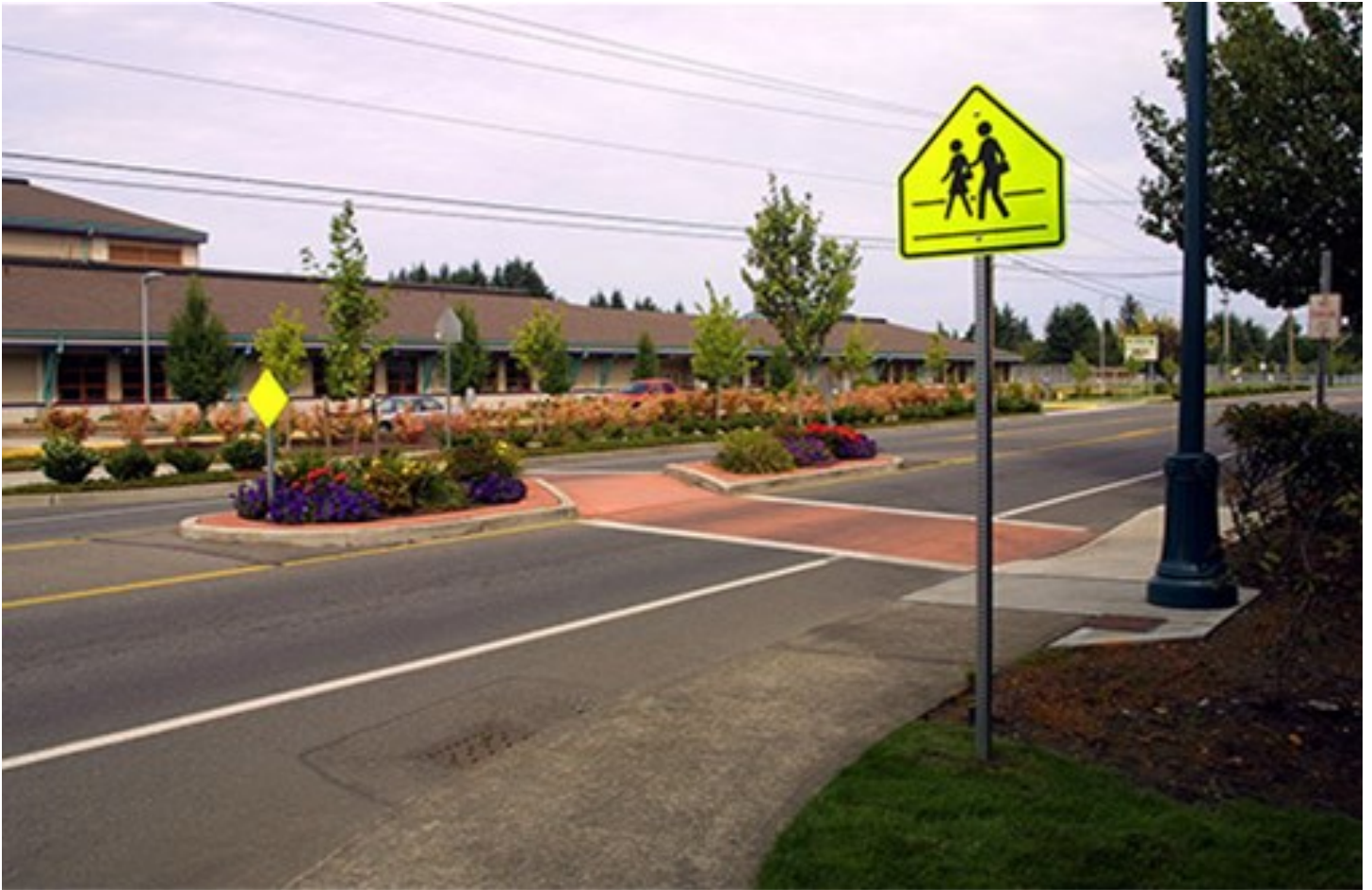
Staggering the crosswalks allows pedestrians to view the oncoming lane before continuing across.
