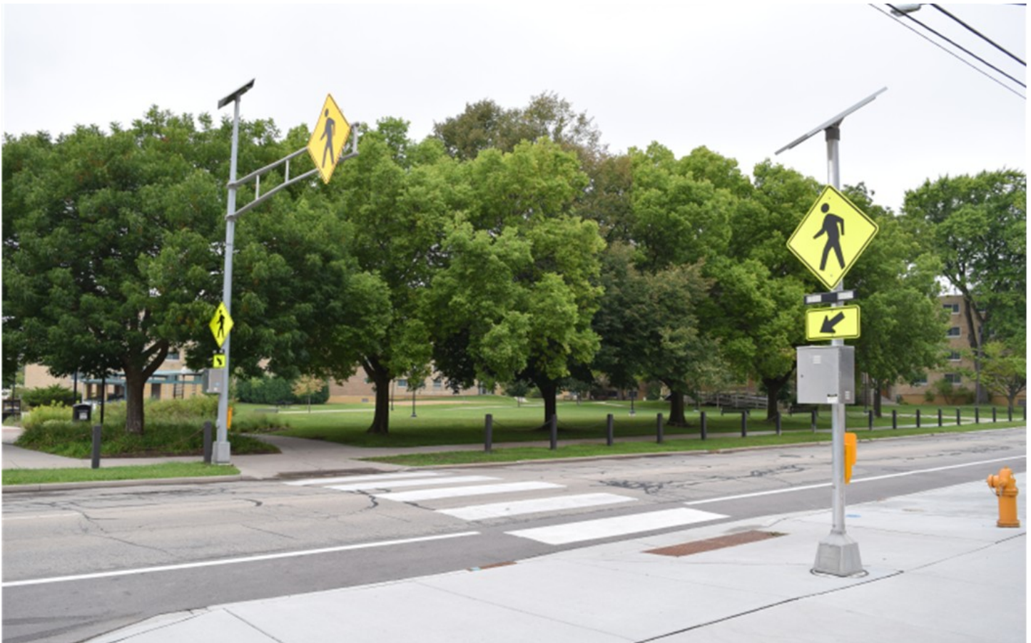
A Rectangular Rapid Flash Beacon announces the presence of bicycle riders using a roadway crossing.
