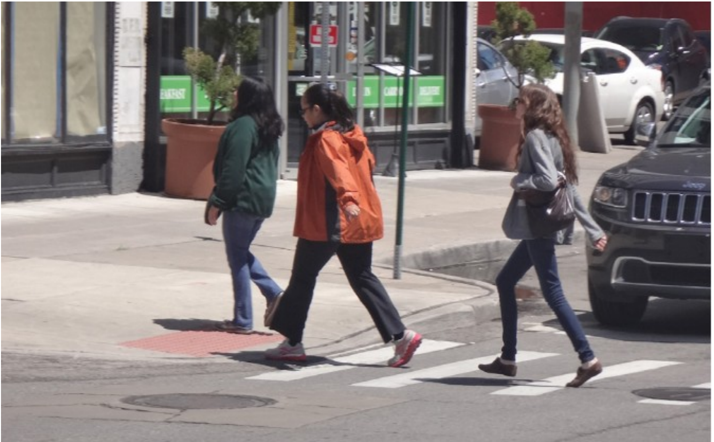
Pedestrian Curb Ramps facilitate access between sidewalk and crosswalk.
