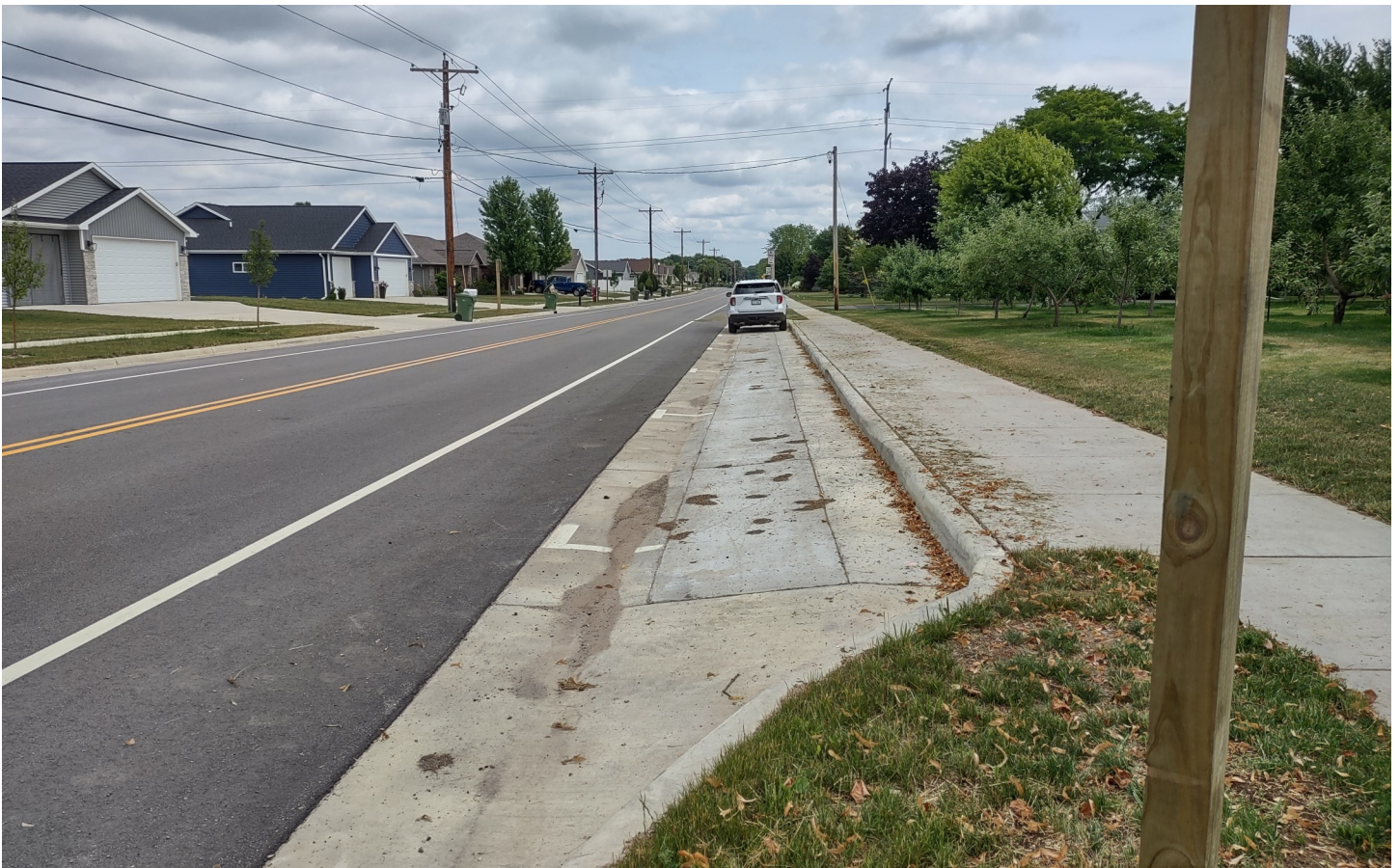
Roadside drop-off and pick-up lanes prevent congestion on the main road, keeping traffic flowing for everyone.
