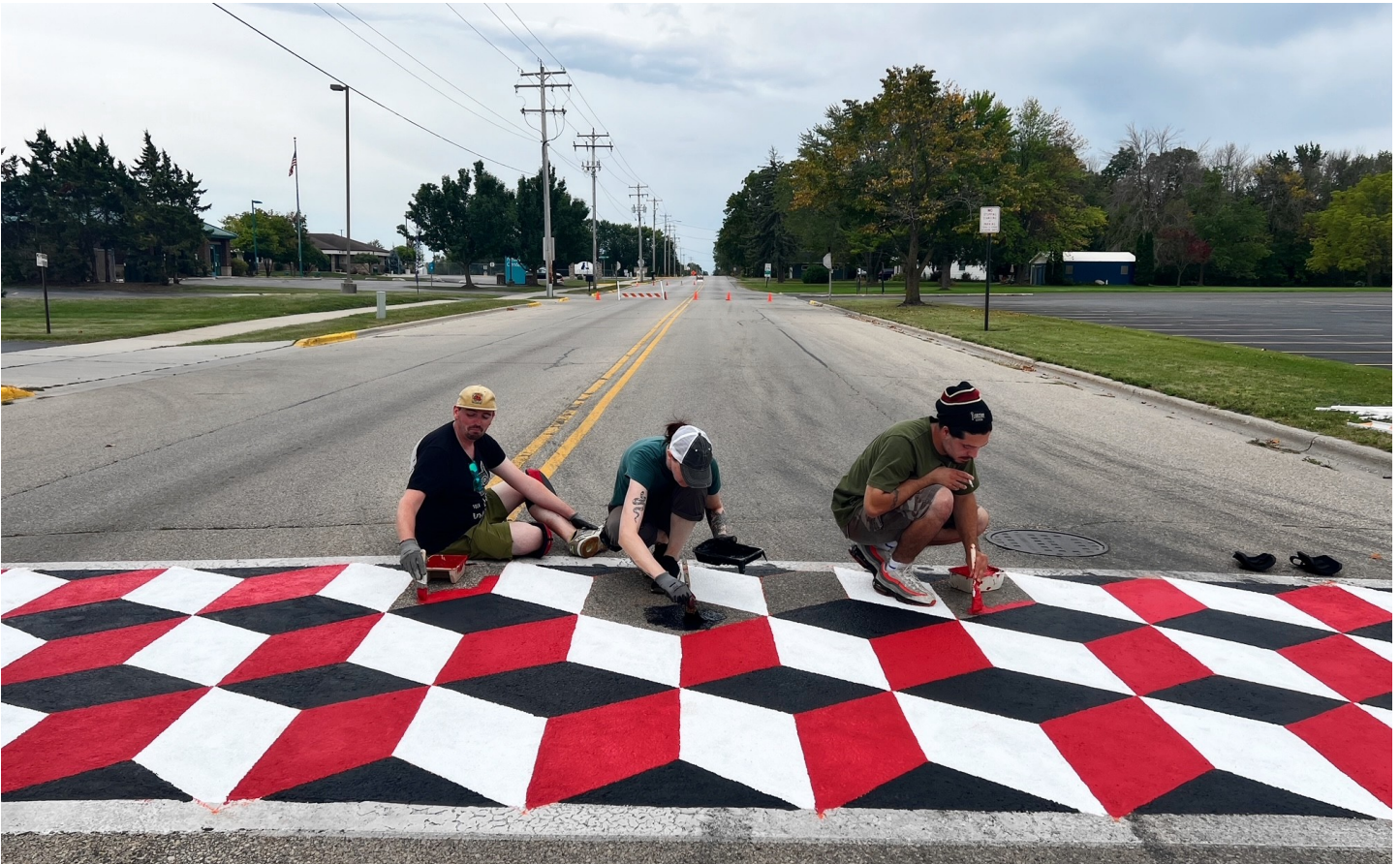
New painted crosswalk at Pulaski Community Middle School.
