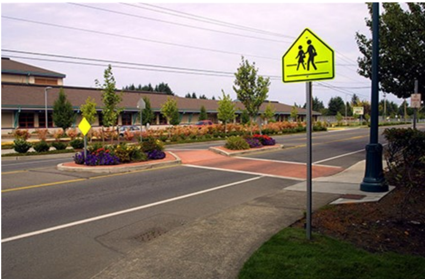
Staggering the crosswalks allows pedestrians to view the oncoming lane before continuing across.
